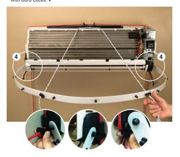
5. Lift the C-Band up into position by pulling White Cords through the Cord Locks. ▼
