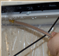
Clean fan blades and blower wheel
